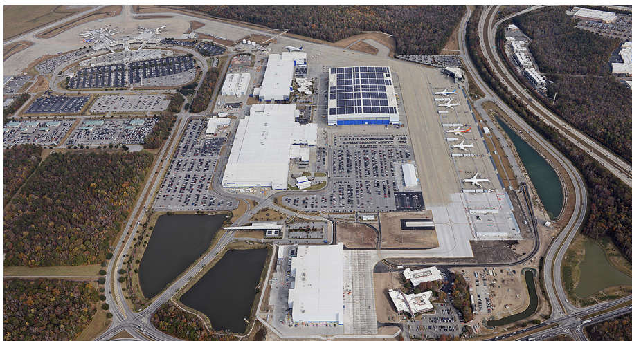
BOEING SOUTH CAROLINA, MAIN CAMPUS, WITH CHARLESTON INTERNATIONAL AIRPORT IN THE BACKGROUND. (SOURCE: WWW.BOEING.COM/COMPANY/ABOUT-BCA/SOUTH-CAROLINA-PRODUCTION-FACILITY EXTRACTED NOVEMBER 22, 2017)
